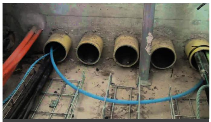
If you are digging a trench to lay fiber then you should be using a blown fiber system so that you can easily replace the fiber in the future. Watch this to see how it works inside the conduit.
